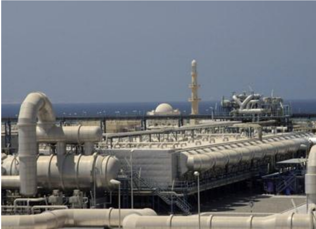
A desalination plant in GCC
